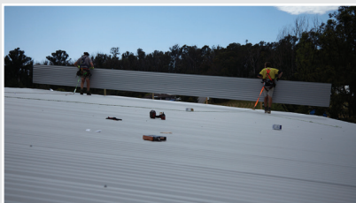
Install roofing onto BuiltQuik frame.
