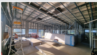
Install ceiling battens and internal walls then run services.
