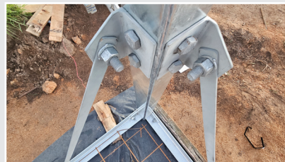
Install bracing to structural plans.
