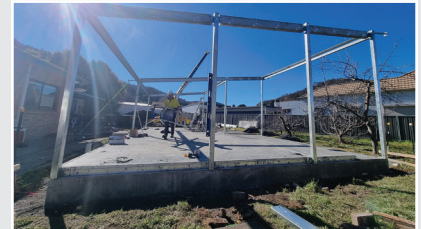
Install rafters and beams.
