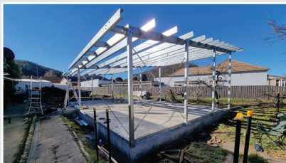
Install roof purlins and eaves.
