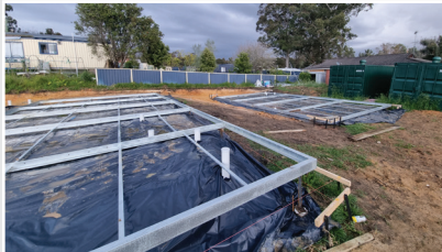
Floor panel installation onto piers.
