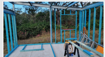
Install external studwork and cladding for lock-up.
